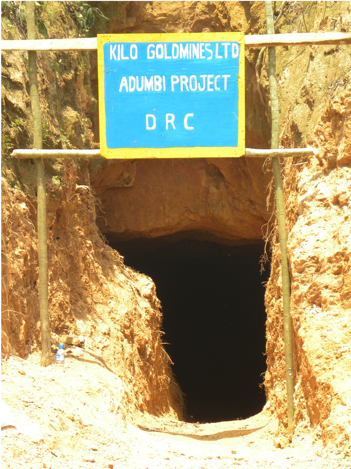
Figure 2) KGL Somituri Project - Adit entrance at the Adumbi site.
